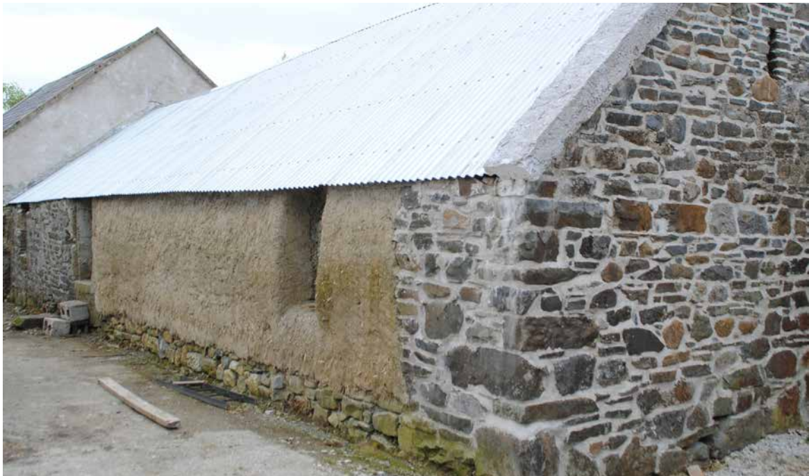
Mud Walled Building, Co Limerick. REPS 4 Traditional Building Grants Scheme - before and after.
