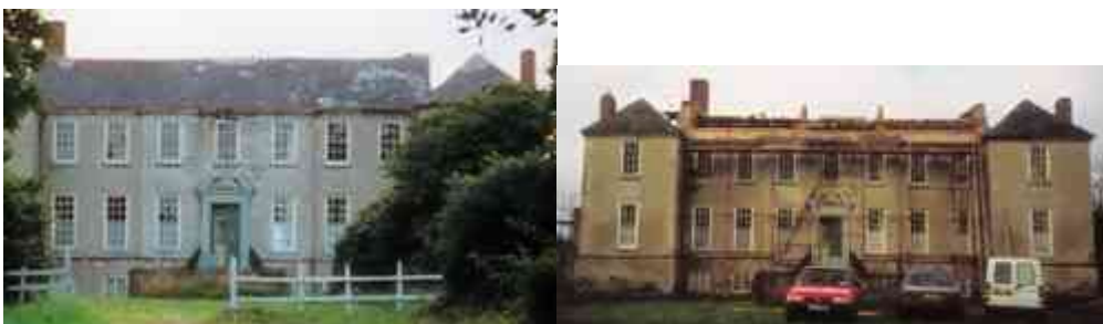
Buncrana "Castle", Co. Donegal, before and during the restoration of the roof of the building
