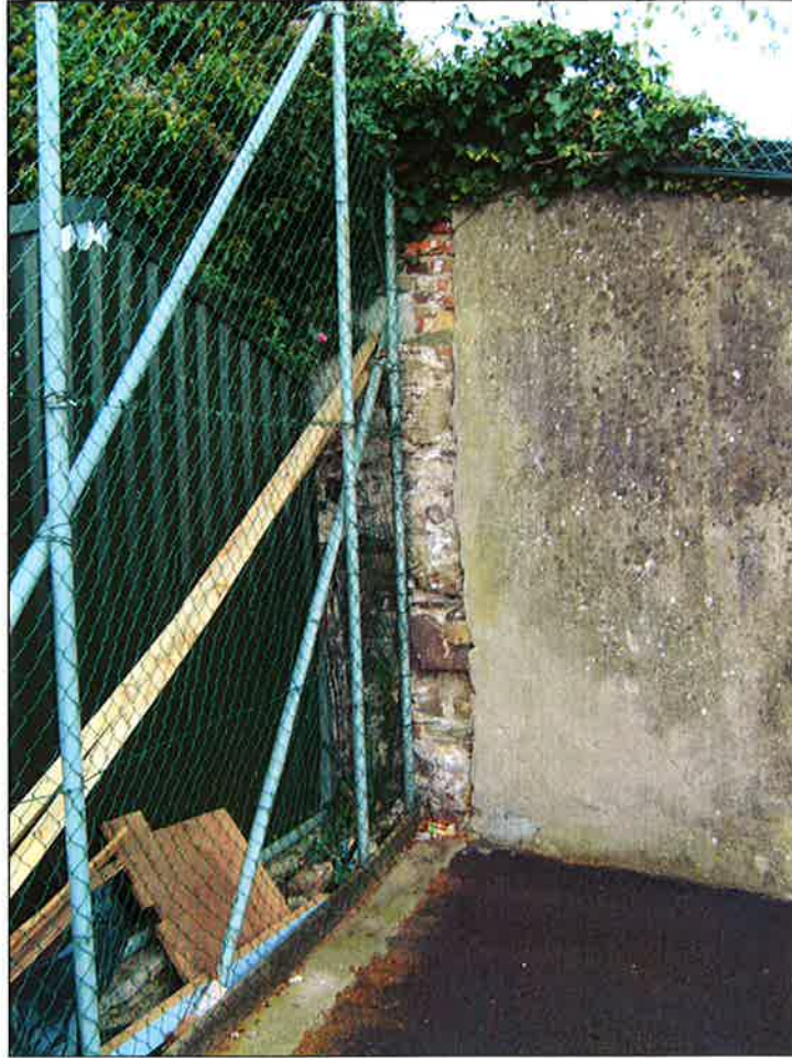
E1 behind garden centre
