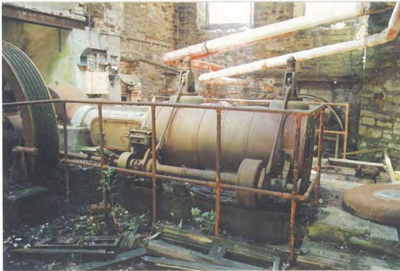
Plate 6: The Robey Uniflow Engine, one of two steam engines installed during the Tannery phase. This is an important piece of the industrial heritage but remains vulnerable through exposure to the elements
