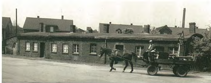
Plate 15: Portlaw roofs on workers' housing at the Mulvany Coal Works, Gelsenkirchen
