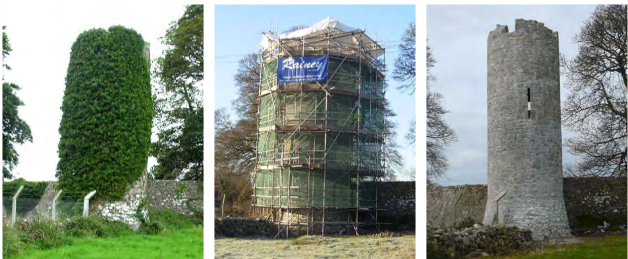
Fig.93 Views of a defensive tower in Athenry before, during and after conservation repairs.
