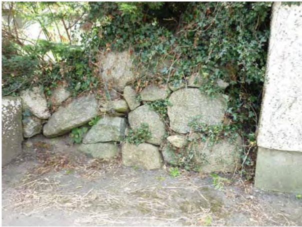
Fig.43 View of large stones loosely laid in retaining wall.
