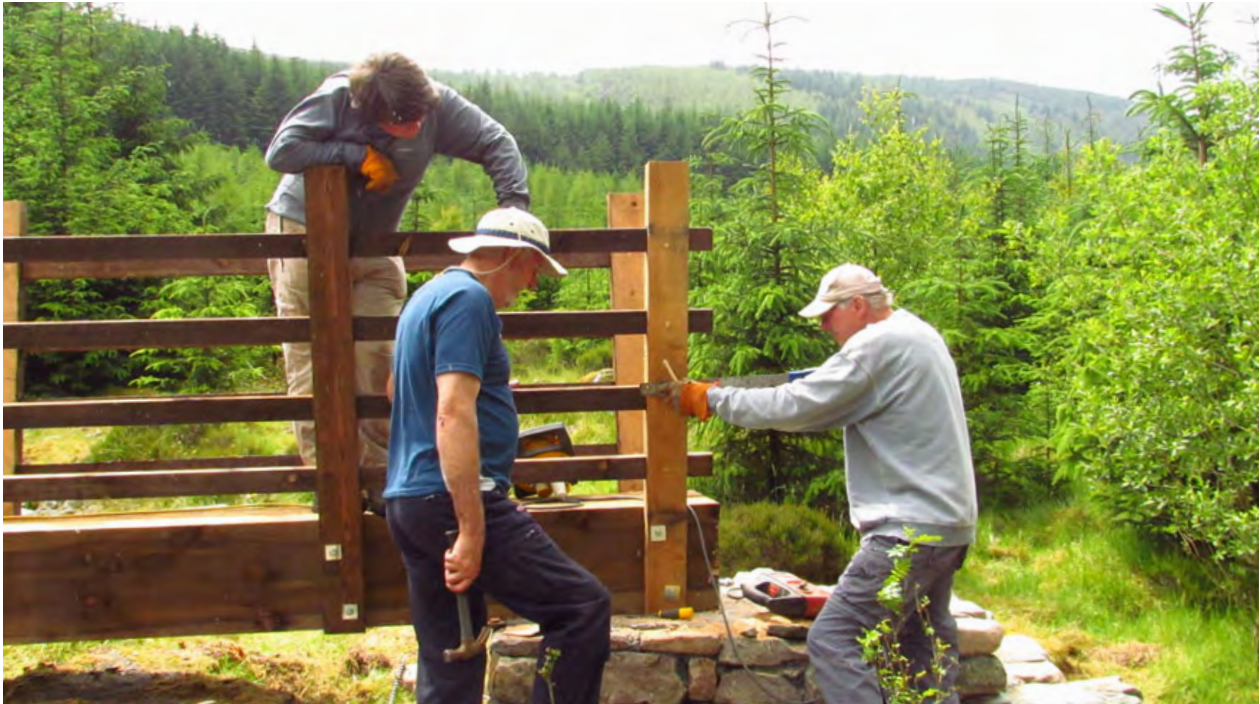
Volunteers repairing a bridge Ennerdale, Lake District, UK (Image: Wild Ennerdale 2025)
