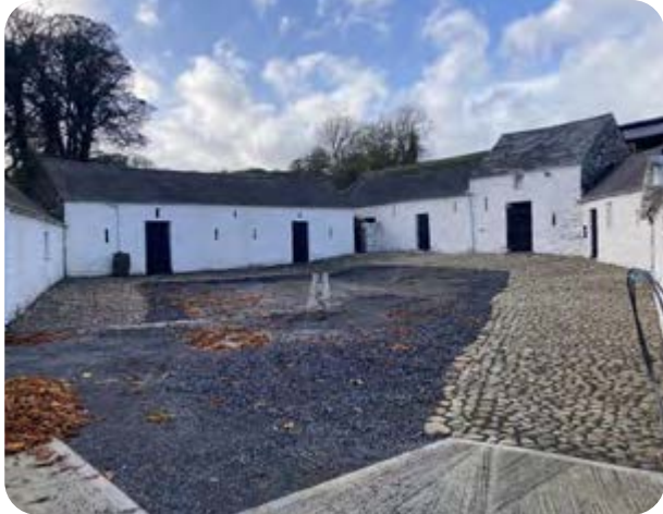
Works carried out on the cobblestone yard in Meath.
