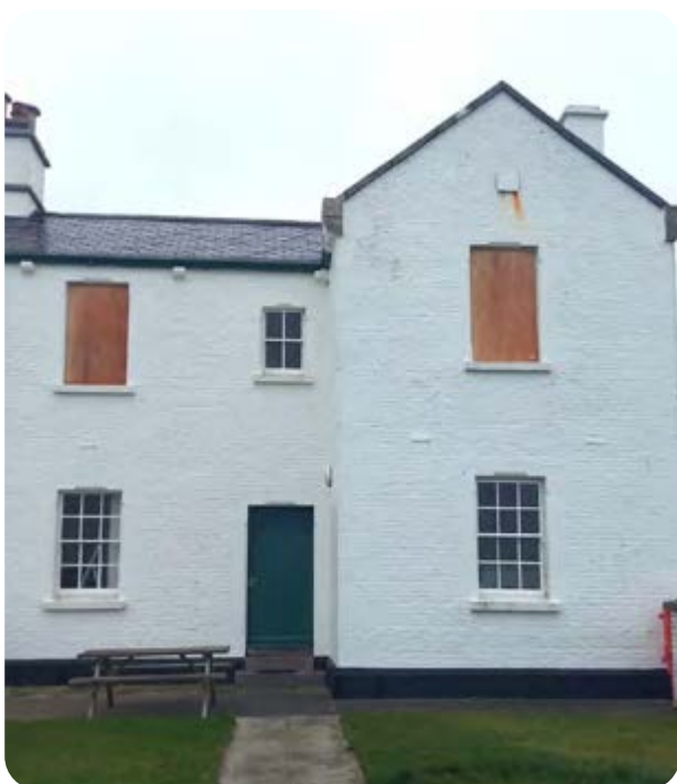
Below right: Galley Head front wall stripped.
