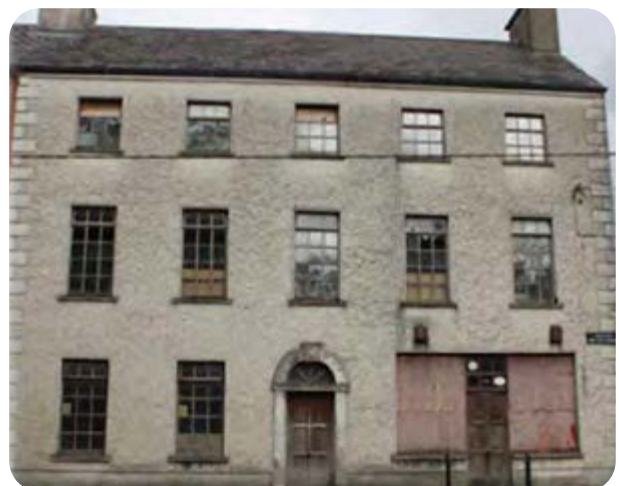
Vacant house and commercial unit, West End Monasterevin. Vacant, at risk.
