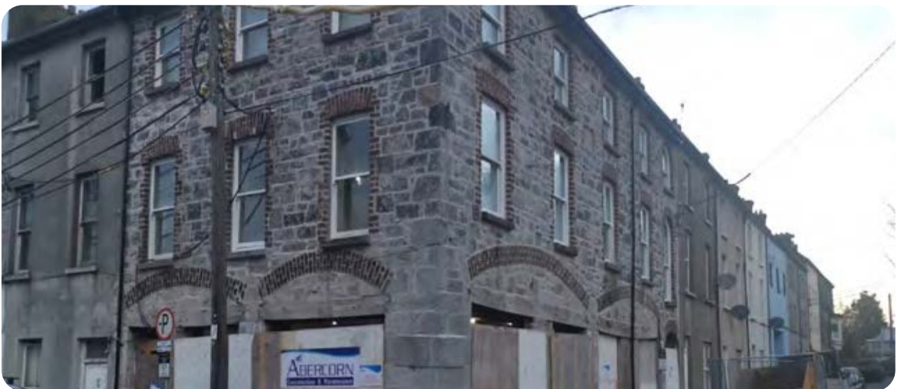
Tipperary Glove Factory before and after completion of conservation works.
