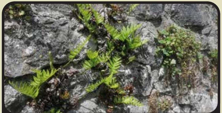
*Toadflax and small ferns do not damage walls. Toadflax in particular merely needs to be kept from growing to an extent where it clogs gutters or obscures possible problems.*
