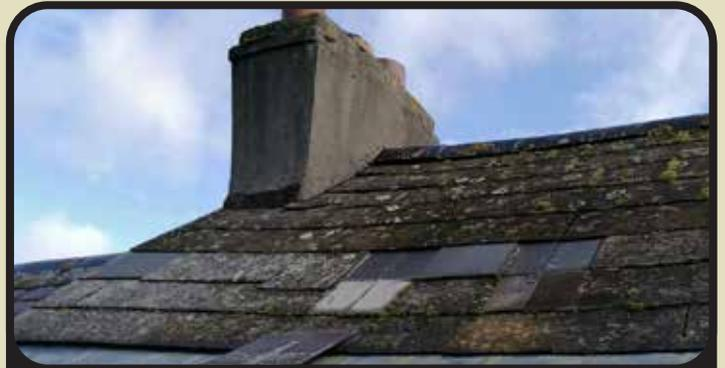
*The missing slates, lack of adequate flashing around the chimney and loss of mortar between ridge tiles were causing several leaks in this roof.*
