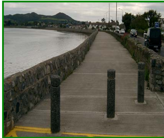
Figure 1. Paved coastal walkway along Fingal coast.
